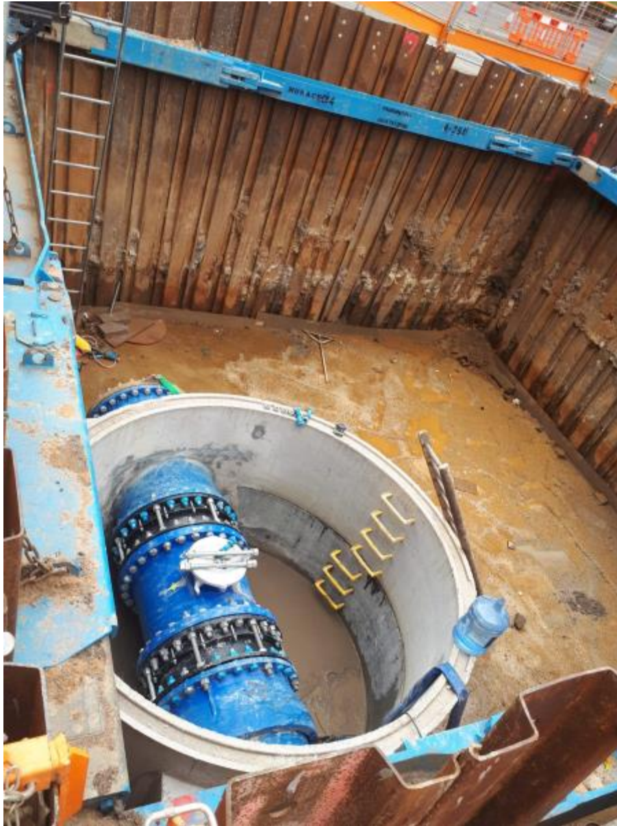
8 - prepping for large valve installation
