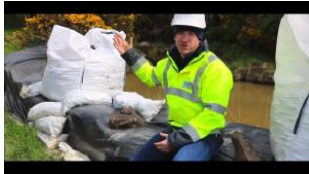
17 - Reservoir refills after investigatory works
