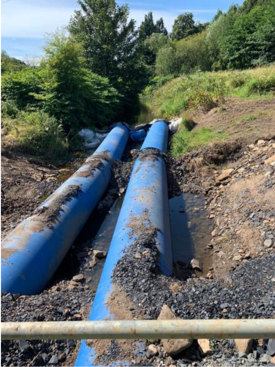
6 - Pipes being installed
